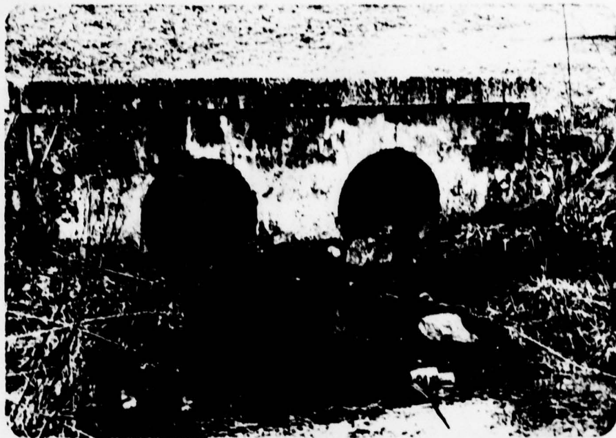
Photograph No. 5 Outlet pipes.
