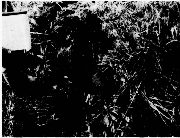
SATURATED GROUND NEAR RIGHT ABUTMENT OF DAM NO. 1
