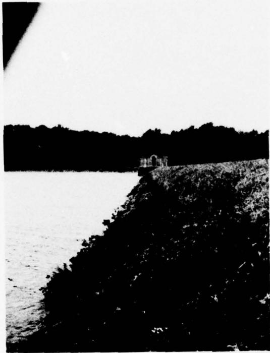
UPSTREAM SLOPE AND CENTER GATEHOUSE DAM NO. 1
