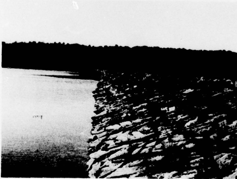
VIEW OF UPSTREAM FACE OF DAM
