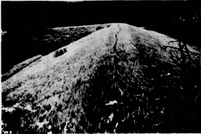
TOP OF EARTHEN BERM VIEW FROM NORTHEAST Photo #1
