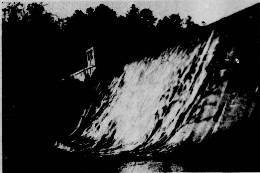
VIEW OF WESTERN SECTION OF DOWNSTREAM SIDE OF SPILLWAY Photo #1
