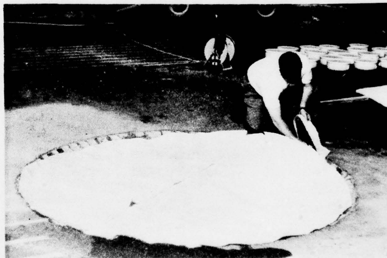
Figure 48. Installation of Fiberglass Cloth in Large Crater
