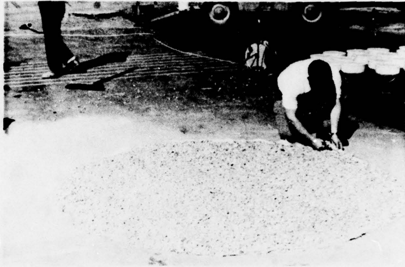
Figure 49. Final Layer of Aggregate in Large Crater
