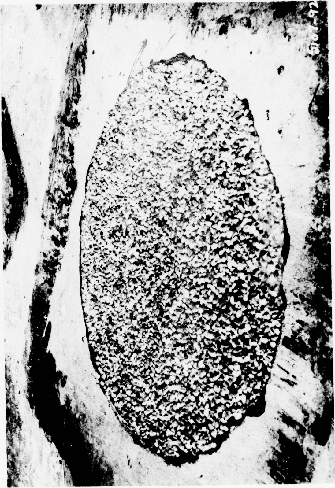
Figure 39. Cured Epoxy Repair Cap
