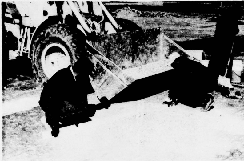
Figure 42. Preparation of Polyester Repair Cap (Intermediate Crater)
