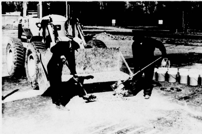
Figure 42. Preparation of Polyester Repair Cap (Intermediate Crater) (Concluded)
