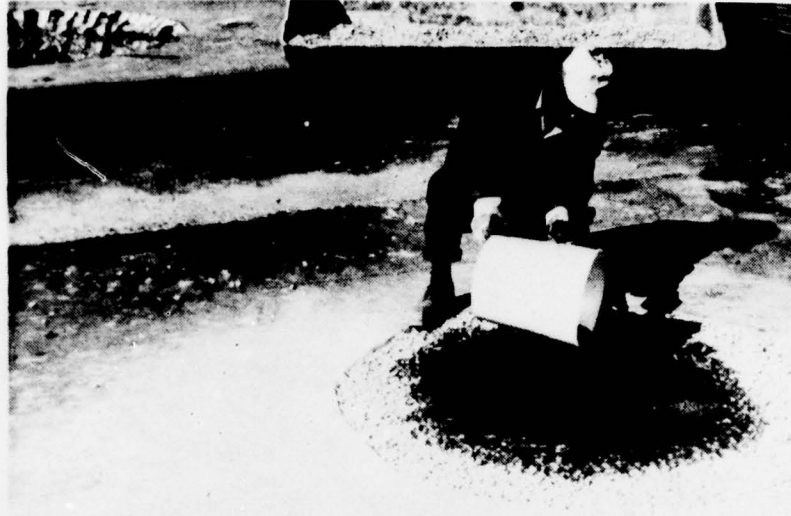
Figure 45. Application of Polyester to Aggregate
