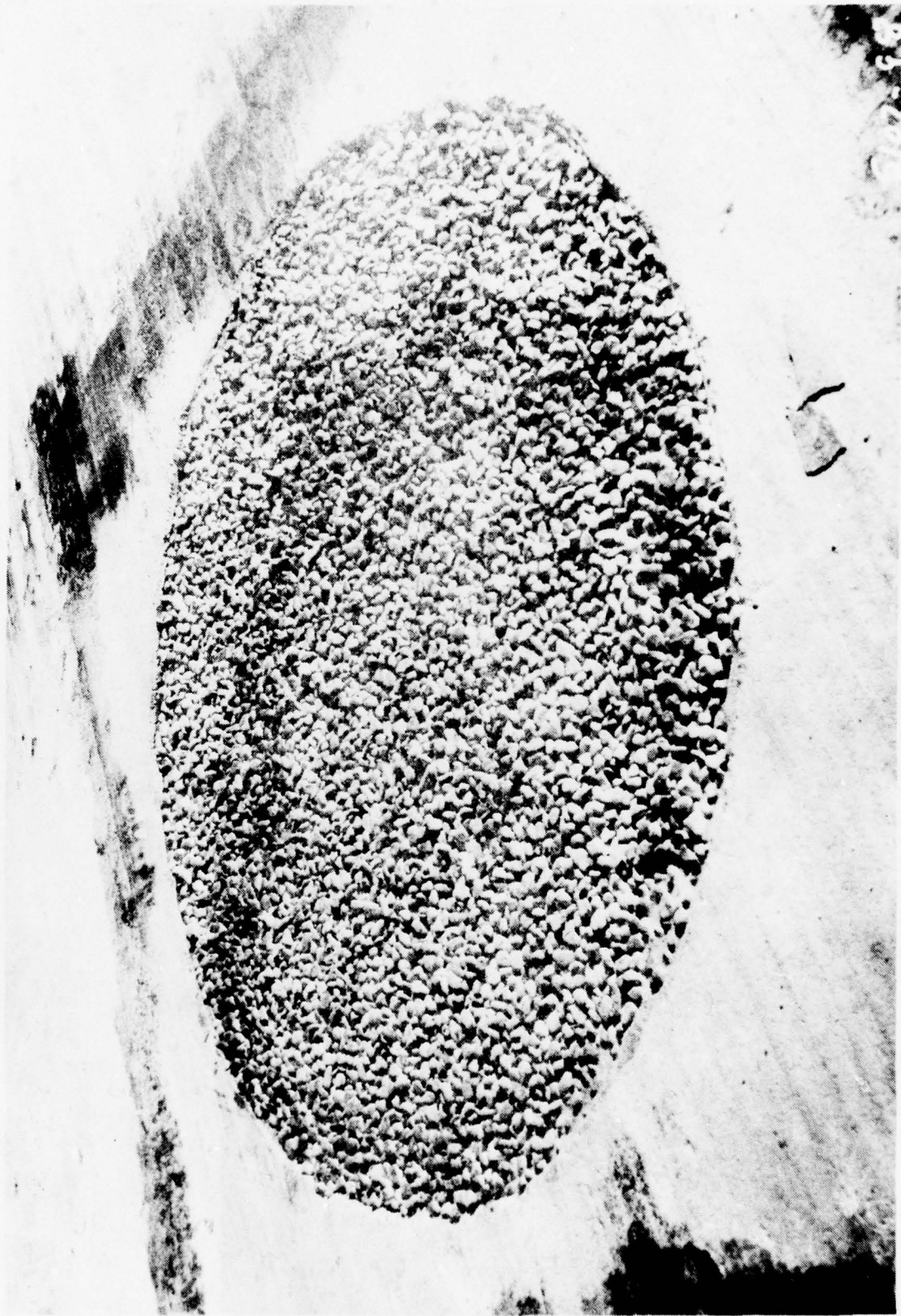
Figure 40. Epoxy Repair Cap After Required Test
