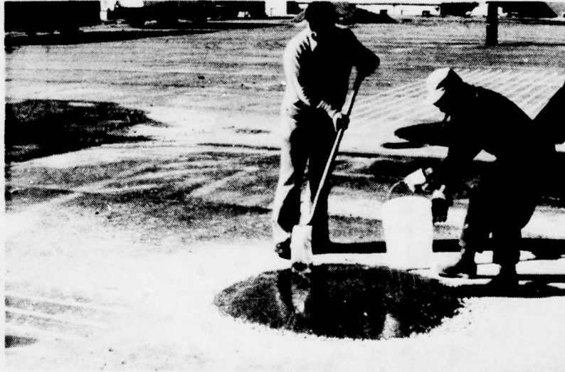
Figure 46. Attempt to Remove Excess Resin
