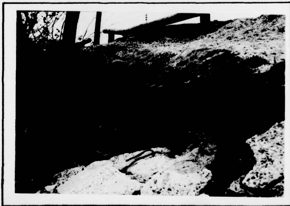
DOWNSTREAM FACE OF THE EMBANKMENT SHOWING EROSION AND MATERIALS INCLUDED IN THE EMBANKMENT D-4
