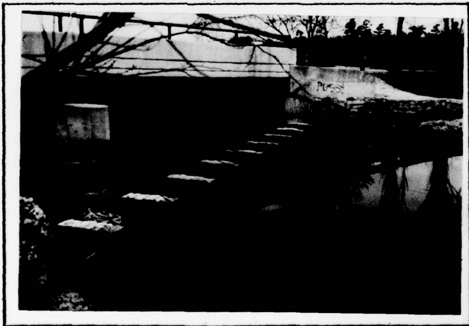
SPILLWAY STOPLOG PIERS AND THE BRIDGE OPENING 4/12/79
