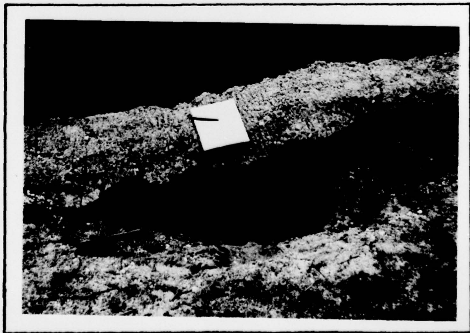
UNDERMINING OF THE BLOCK WALL ALONG THE UPSTREAM EMBANKMENT SLOPE 4/12/79
