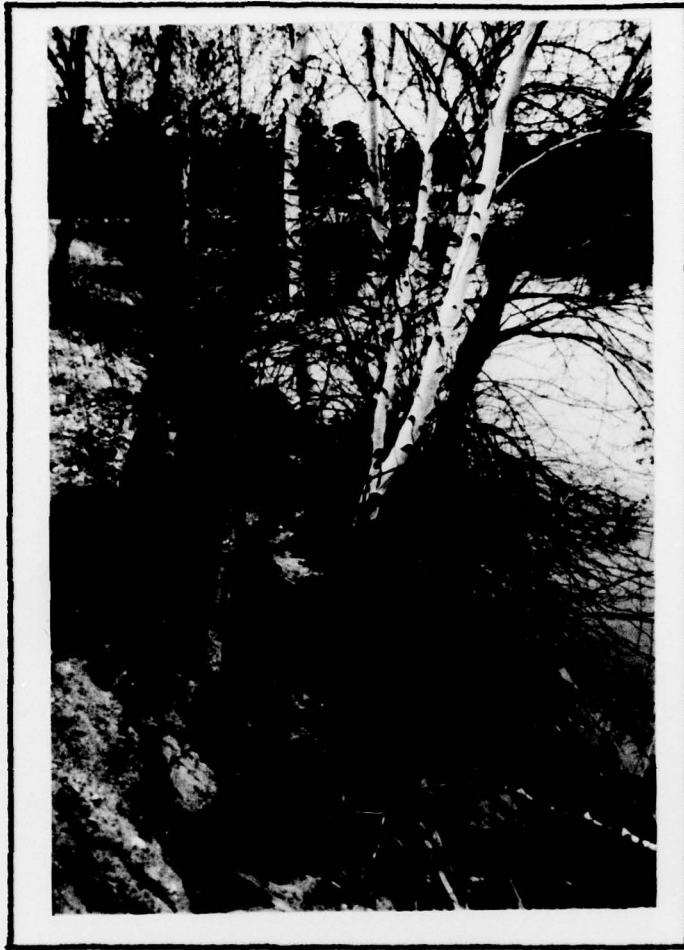
DOWNSTREAM FACE OF THE EMBANKMENT SHOWING DEBRIS AND TREES 4/12/79
