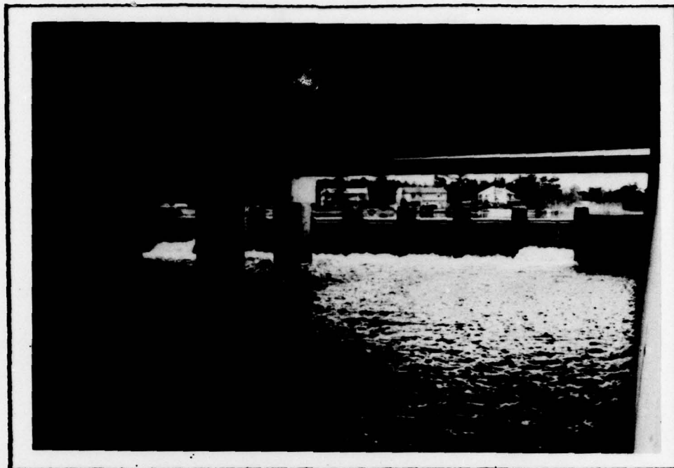
VIEW OF THE BRIDGE OPENING AND THE SPILLWAY STOPLOG PIERS 4/12/79
