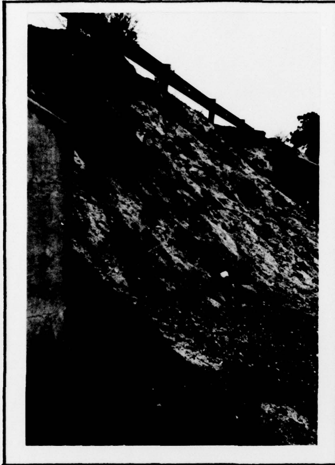
DOWNSTREAM FACE OF THE EMBANKMENT SHOWING EROSION AND LACK OF COVER 4/12/79
