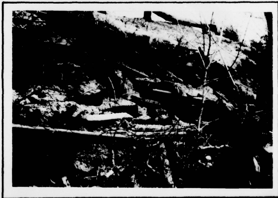
DOWNSTREAM FACE OF THE EMBANKMENT SHOWING EXTENSIVE DEBRIS 4/12/79
