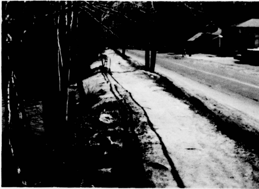
PHOTO 1 CREST OF DYKE
