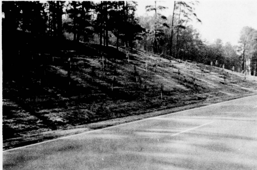
Landscape view on south lane of Benning Boulevard. Pines were planted on steep slopes for beauty and to reduce mowing in this area.
