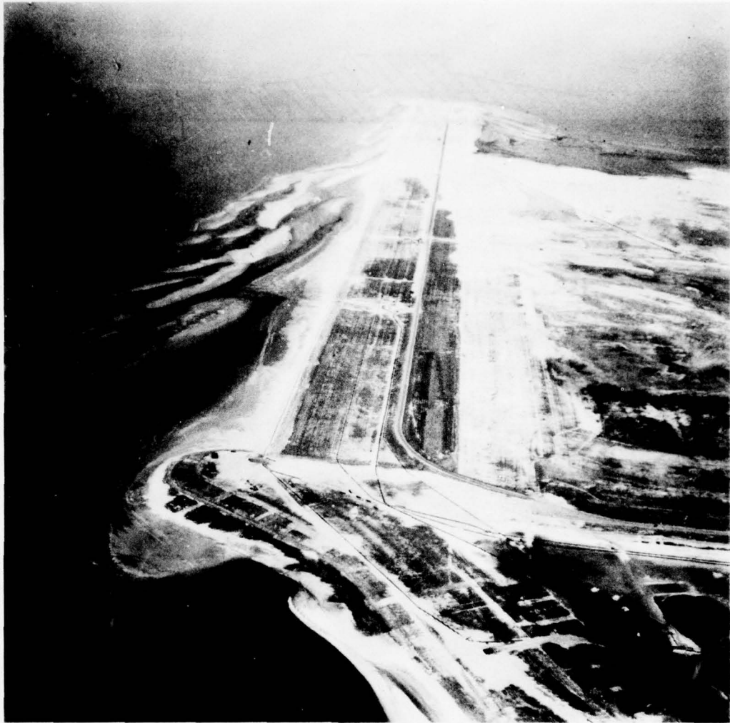
Figure 25. Aerial view of sand dam in Europoort consisted of sand with a diameter from 150 to 250 \mu . This resulted in underwater slopes of the dam in the order of 1:10 to 1:60, depending upon grain size (Figure 27). Later on the slopes flattened out to 1:50. The sand was dredged by means of plain suction dredges from a depth of up to 40 m below sea level. The work was carried out by two suction dredges with a combined output of approximately 3000 \text{m}^3 of sand per hour (104 hours per week) and a mixture density on the order of 1250 \text{kg}/\text{m}^3 . The total amount of sand in the dam amounts to approximately 35 million \text{m}^3 . At present, the outer slope is used as a recreational
