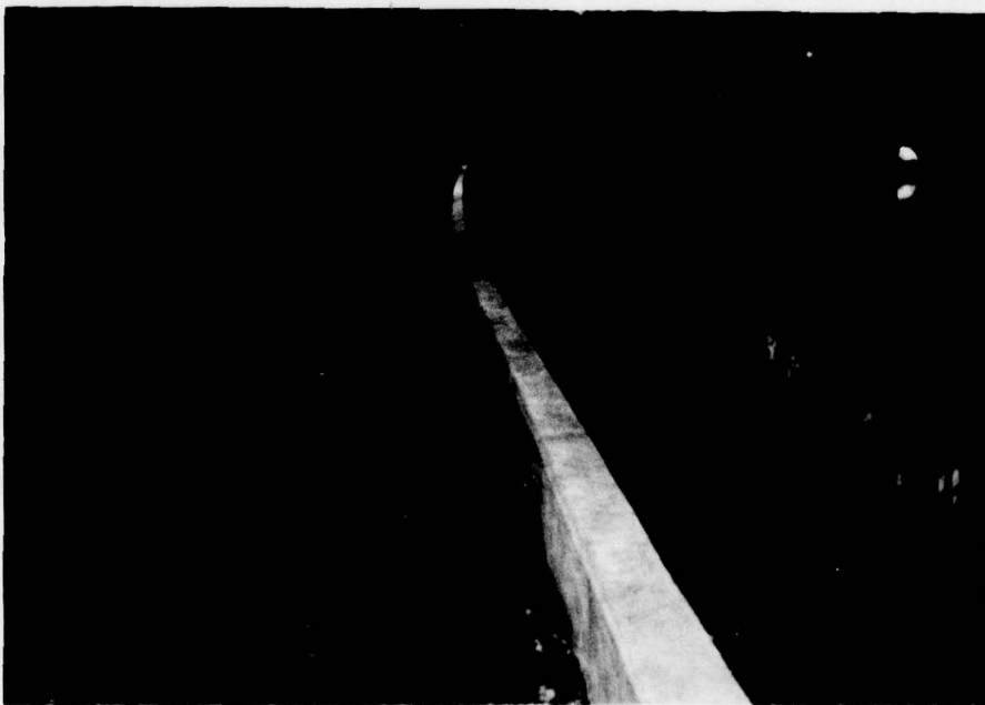
PHOTO 4 CREST OF DAM
