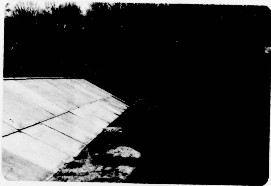
View of Primary Spillway Outlet
