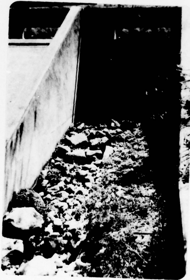
View of Sluiceway Outlet Channel
