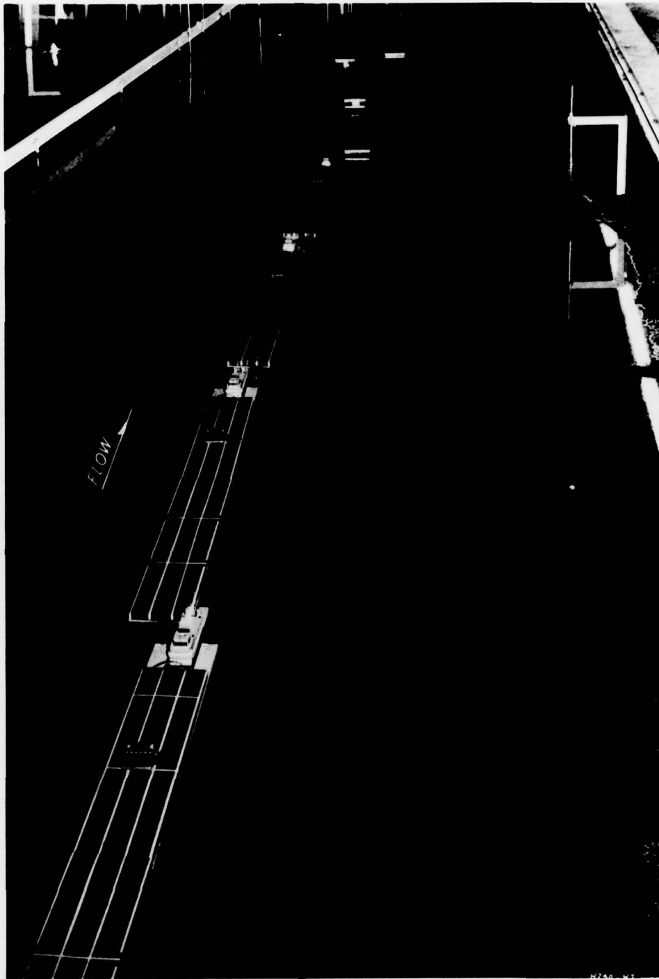
Photo 5. Plan B. Discharge 203,000 cfs; upper pool el 294.4. Path of upbound tow leaving the riverside lock
