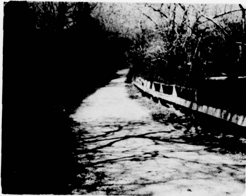
View of Crest
