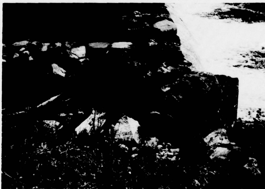
PHOTO 2 WASHOUT ADJACENT TO NORTH END OF SPILLWAY
