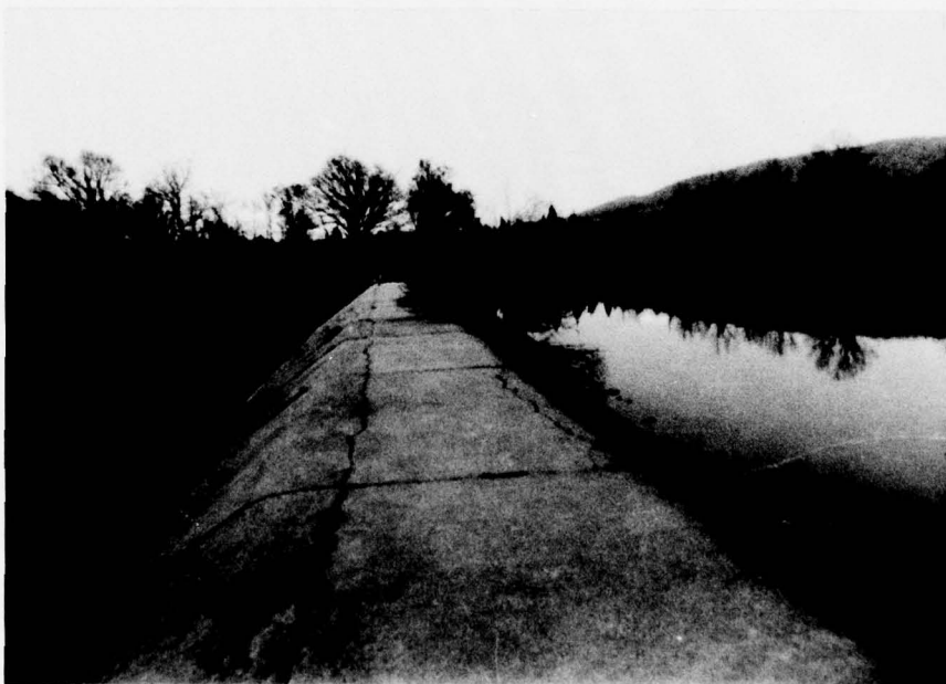
Photo No. 5 - View of left embankment looking towards the spillway. Note that toe protection has been provided along the length of the embankment.
