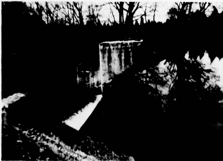
Photo No. 1 - Overall view of spillway from left side. The foot-bridge has been removed. Note the key shaft for the low level outlet valve in the central buttress, and the advanced deterioration of the concrete at the water line.
