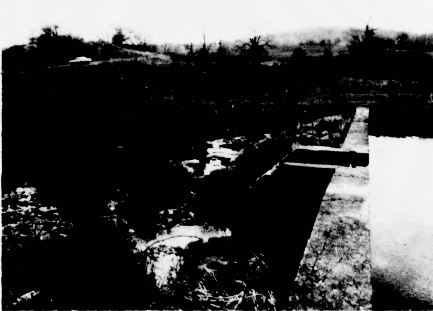
Photo No. 10 - Retaining structure of downstream pond.
