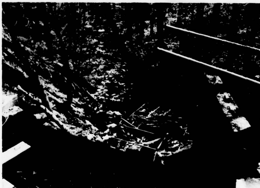
Photo No. 8 - Overall view of downstream channel from top of dam. showing spillway in foreground. Note the steep, wooded valley sides, and the debris in the channel.
