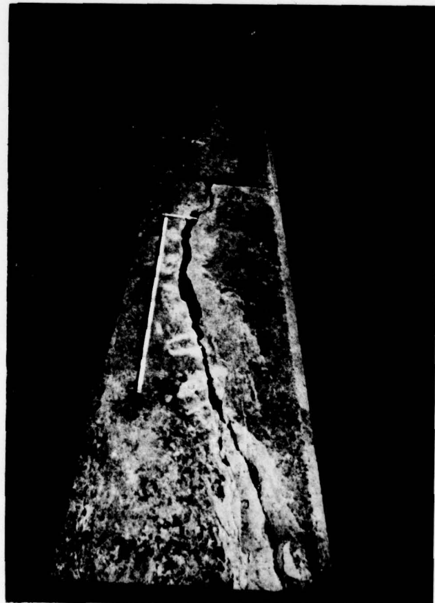
Photo No. 8 - Detail showing the movement crack in the right wingwall, upstream of the footbridge.
