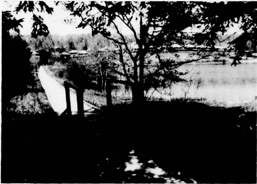
Photo No. 3 - View of concrete walkway along the crest and the emergency spillway. Note outlet pipe from the lake.
