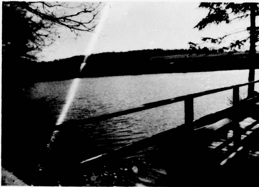
Photo No. 7 - Overall view of reservoir from spillway bridge, looking upstream.
