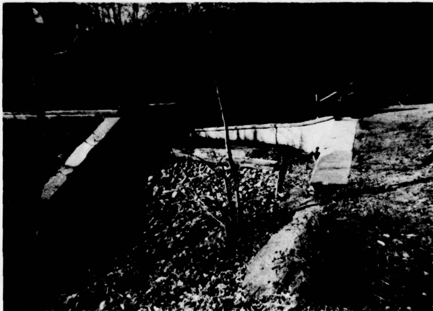
Photo No. 2 - Overall view of upstream face of spillway. Note build-up of stones and silt at the spillway inlet.
