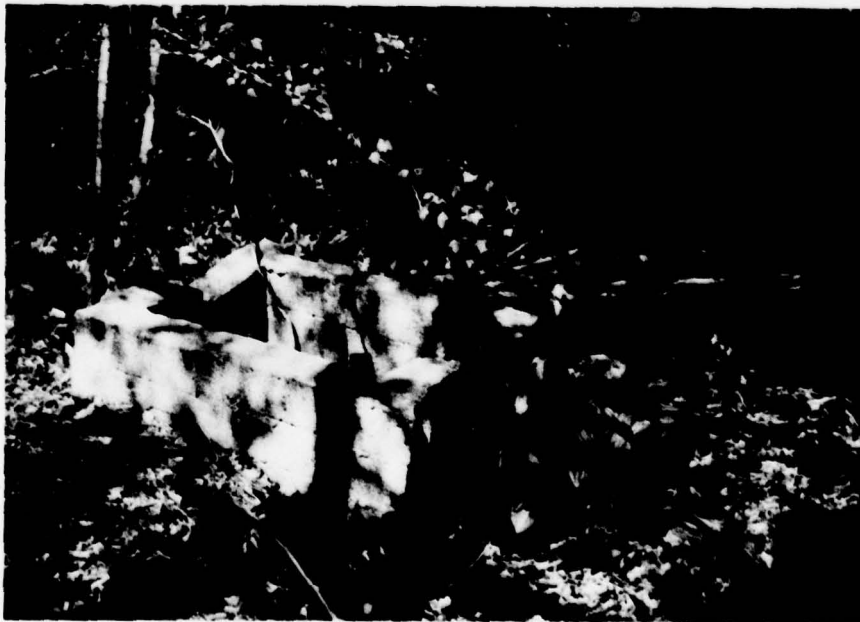
Photo No. 8 - View of observation well approximately 20' below the embankment crest. Note discolored seepage in the surrounding area.
