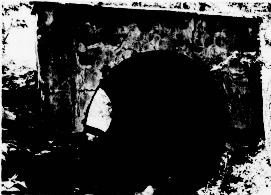
Photo No. 7 - View of 5 foot diameter Armco discharge culvert from the pond. Note deteriorated and cracked headwall. Headwall at other end has partly collapsed. The culvert drains directly onto the embankment face.
