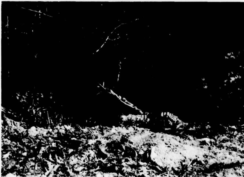
Photo No. 10 - View of washed out area on the downstream face at the turn in the road. Note fallen trees and debris in the area.
