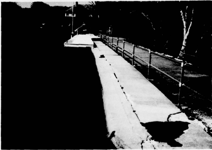
PHOTO 4 UPSTREAM FACE OF DAM
