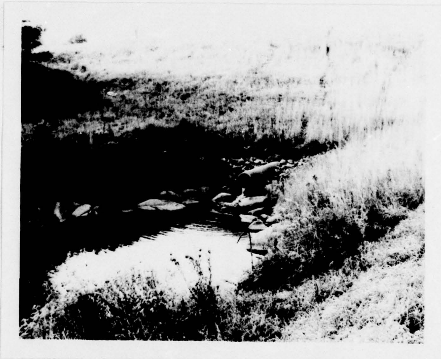
PRINCIPAL SPILLWAY OUTLET PIPE AND PLUNGE POOL (LOOKING UPSTREAM)
