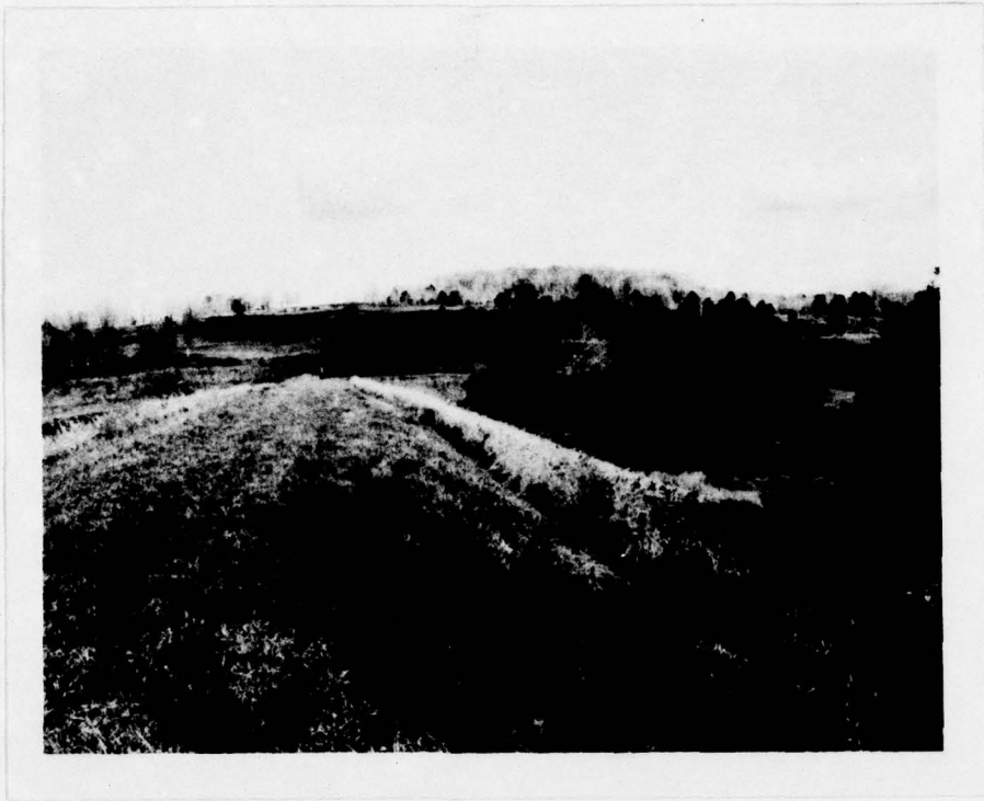
VIEW LOOKING EAST ALONG DAM CREST
