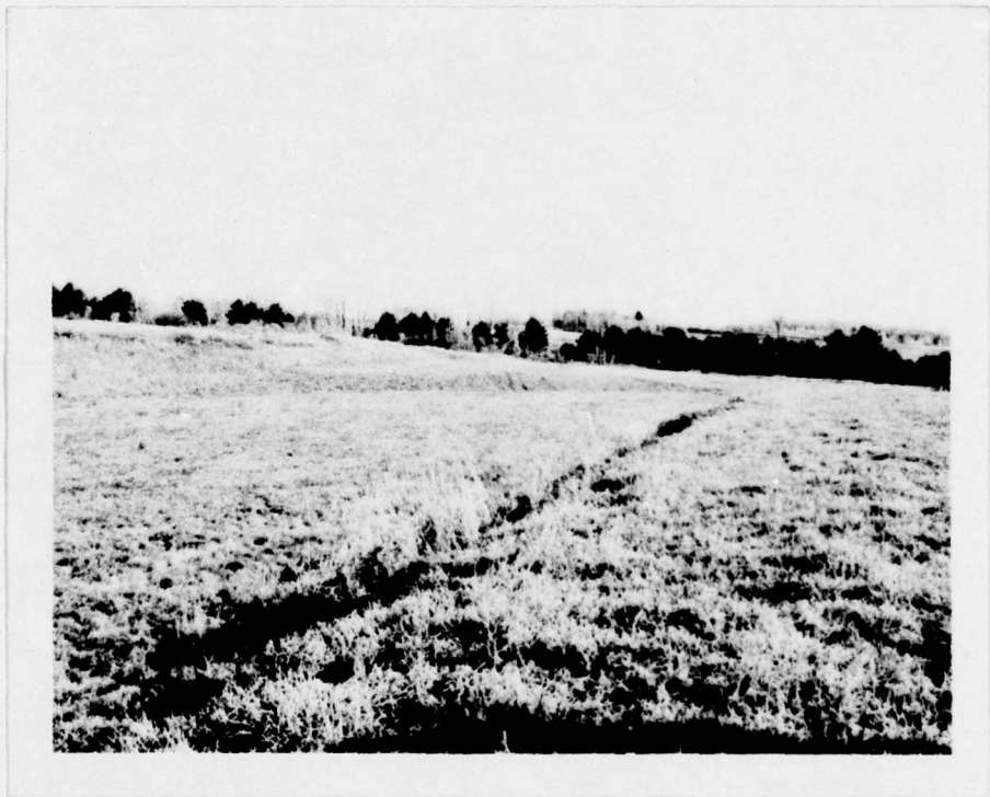
EMERGENCY SPILLWAY LOOKING DOWNSTREAM
