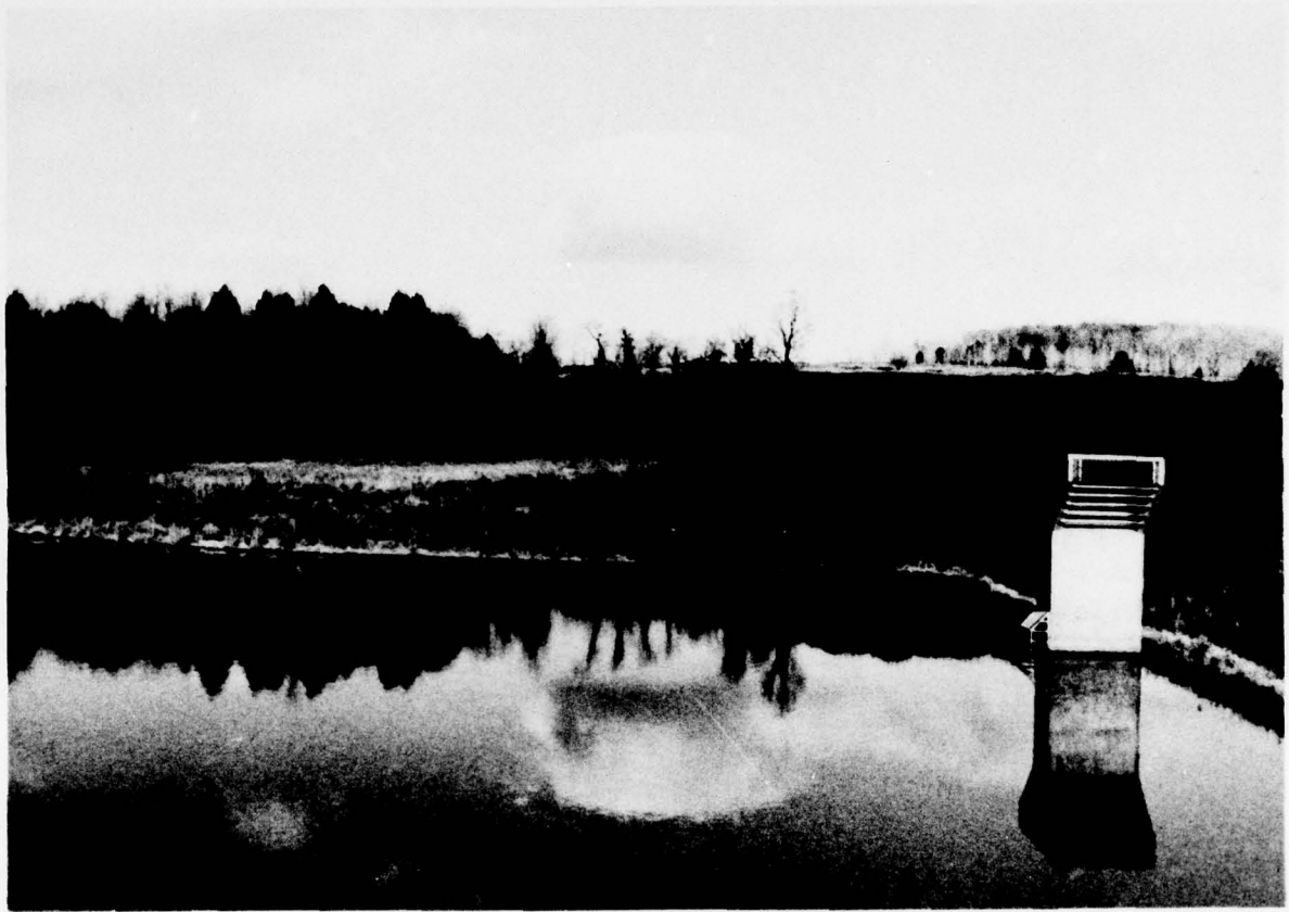
NANTICOKE CREEK SITE No. 8 OVERVIEW NORTHERN END OF UPSTREAM FACE AND EMERGENCY SPILLWAY
