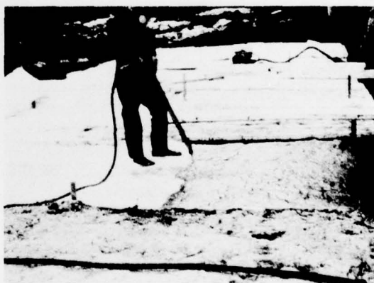
Figure 7. Applying LP-3 modified sulfur foam onto fiberglass mat, May 1971.
