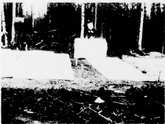
Figure 6. Laying fiberglass mat on frozen substrate, May 1971.
