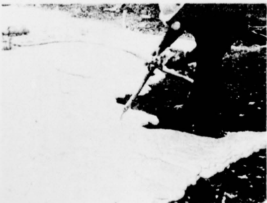
Figure 8. Foam application on frozen substrate of rear half of pad, May 1971.
