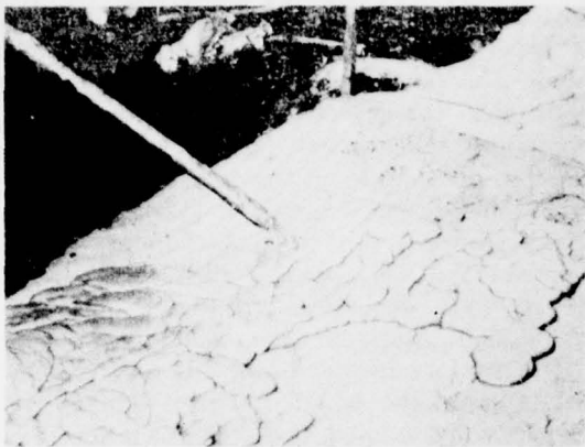
Figure 4. Finish application of foam, showing consistency and application technique, May 1971.
