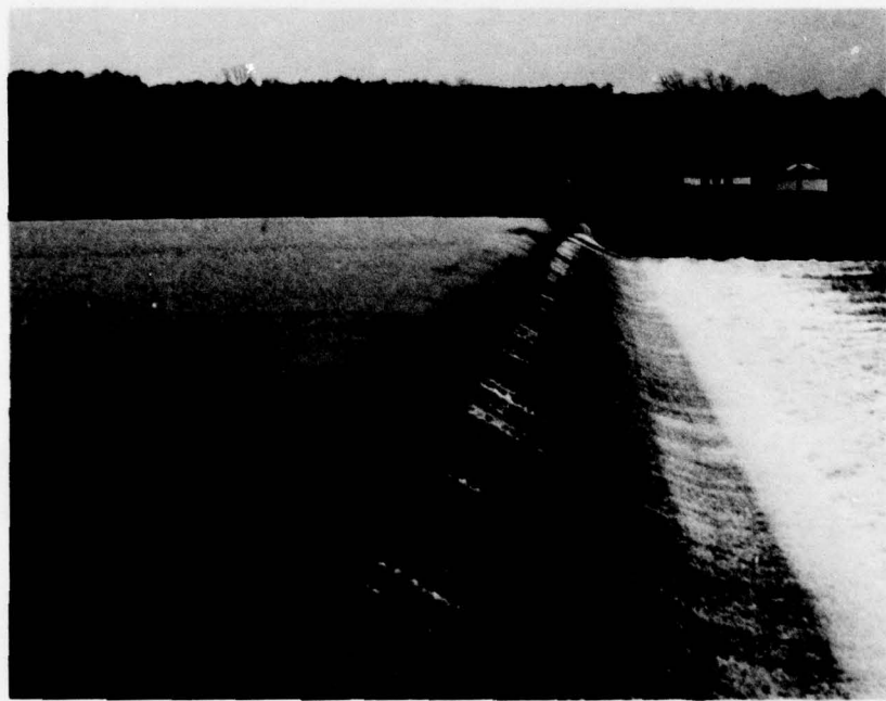
LOCK 3 DAM @ MECHANICVILLE (Looking East)
