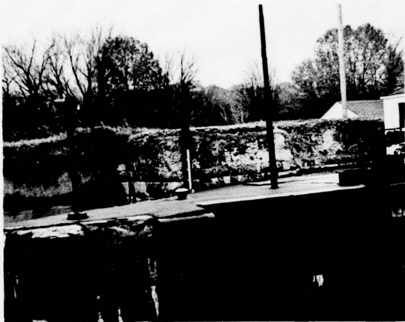
CONCRETE DETERIORATION @ ABUTMENT OF EARTH DIKE - LOCK 3
