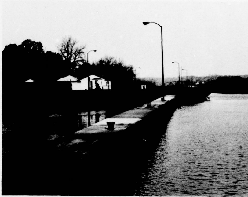
UPSTREAM APPROACH TO LOCK 3
