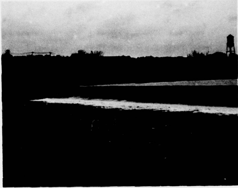
LOCK 3 DAM @ MECHANICVILLE (Looking West)
