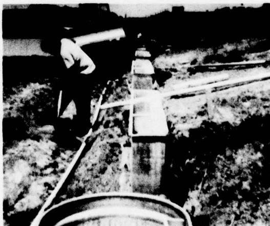
Figure 19. Replacing the sedimentation tanks with underdrains.
