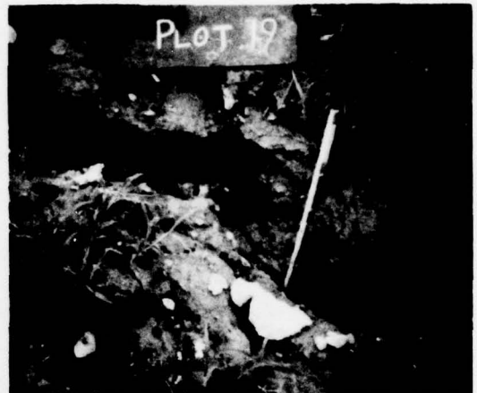
Figure 15. Closeup of damage showing extent of erosion.
