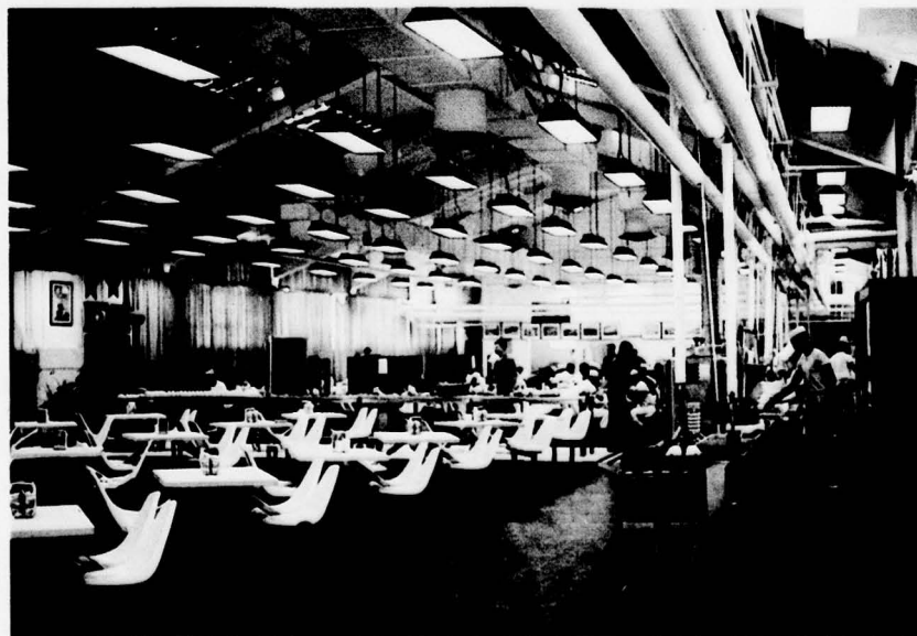
View of the prerenovation condition of the total interior. Note exposed serving line steam piping and ceiling light fixture chains. All users are able to see all others in the entire dining hall at all times.
