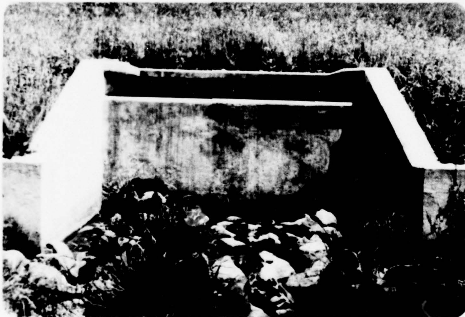
PHOTO #2 OUTLET STRUCTURE
