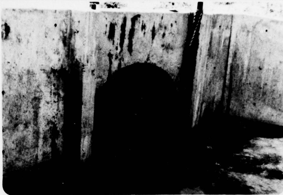
PHOTO # 3 EMERGENCY SPILLWAY
