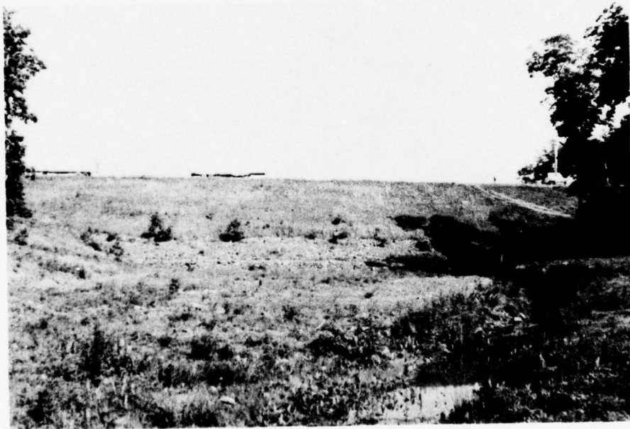
Downstream Face of Dam
