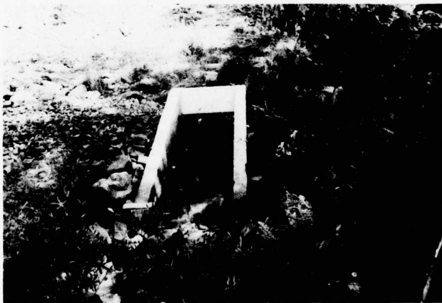
PHOTOGRAPH NO. 2 Discharge Box Culvert
