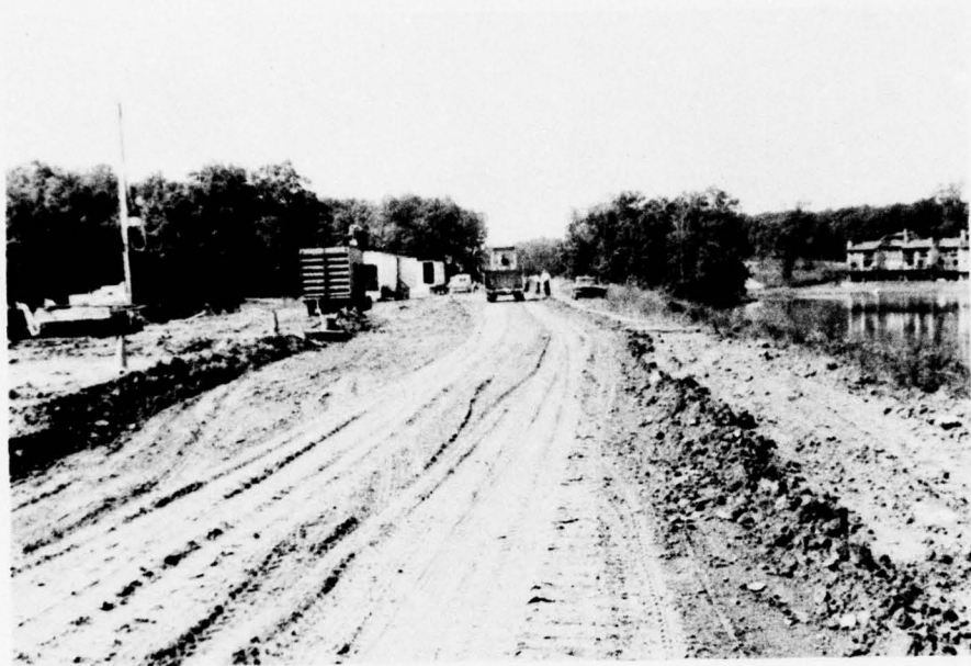
Top of Dam
