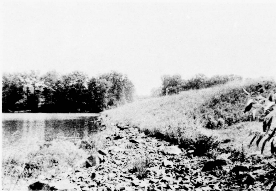
PHOTOGRAPH NO. 3 Upstream Face of Dam
