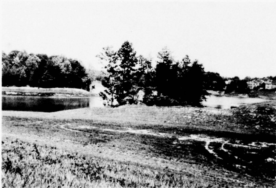
PHOTOGRAPH NO. 2 Emergency Spillway Channel
