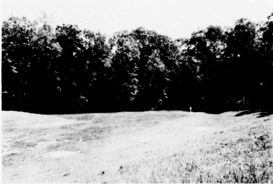
PHOTOGRAPH NO. 3 Emergency Spillway Outlet
