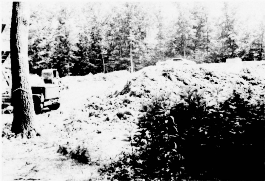
PHOTOGRAPH NO. 4 New Construction Site Adjacent to Emergency Spillway
