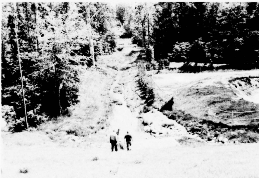
PHOTOGRAPH NO. 6 Downstream
