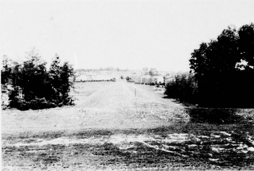
Top of Dam
