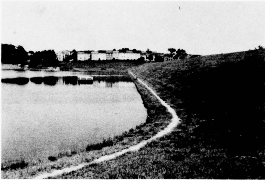
PHOTOGRAPH NO. 1 Upstream Face of Dam and Principal Spillway Intake Structure
