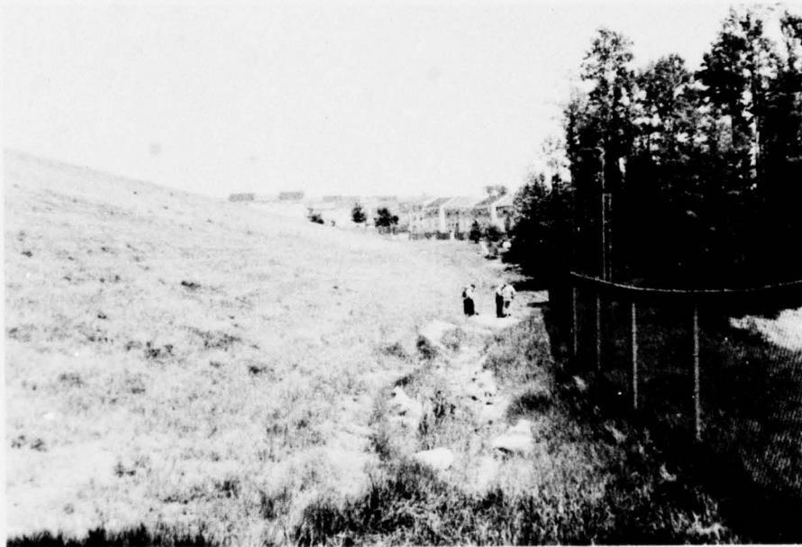
Downstream Face of Dam and Toe Drain
