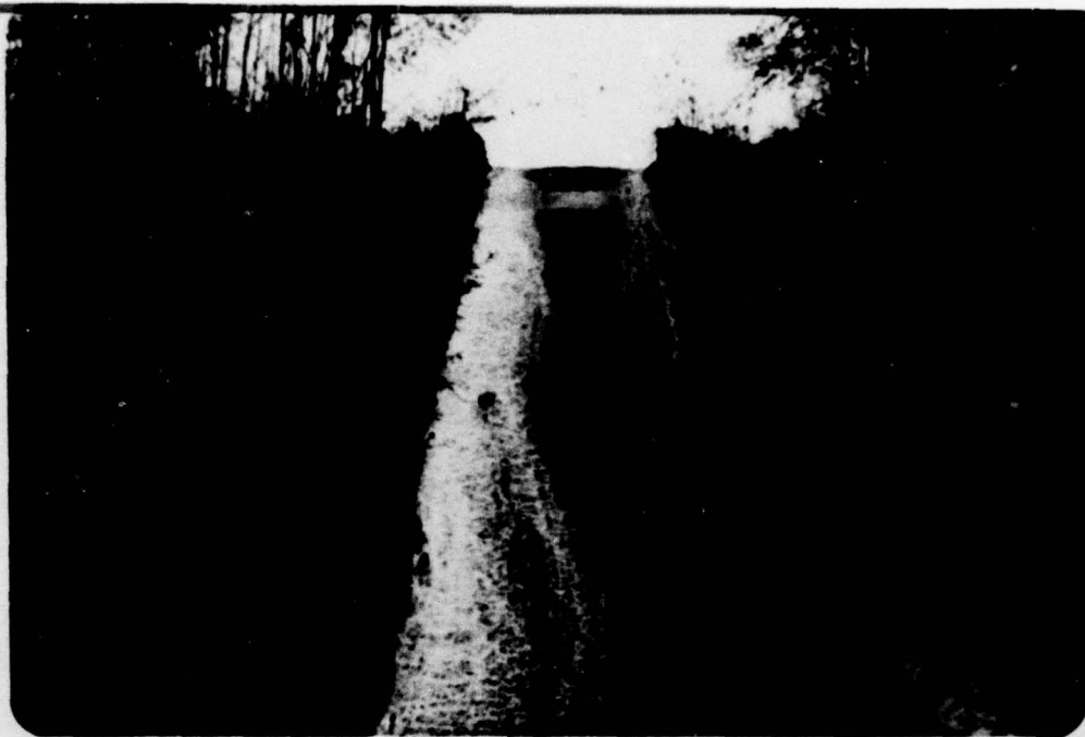
PHOTO # 3 DISCHARGE CHANNEL
