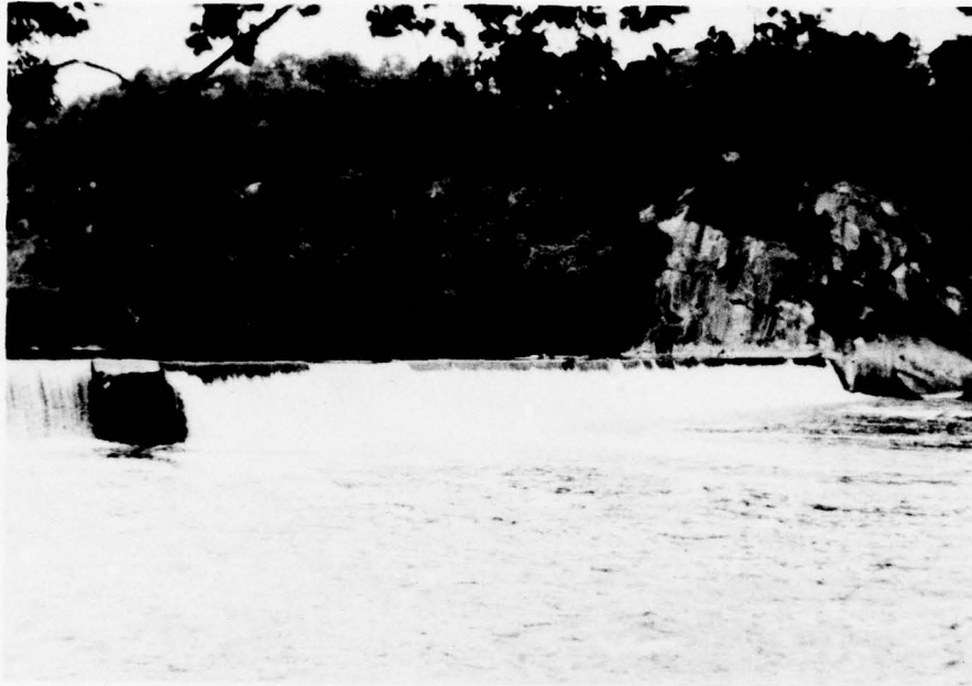
PHOTOGRAPH NO. 1 Spillway
