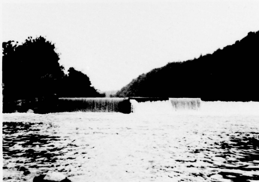
PHOTOGRAPH NO. 2 Front View
