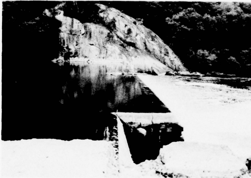
PHOTOGRAPH NO. 2 Left Abutment
