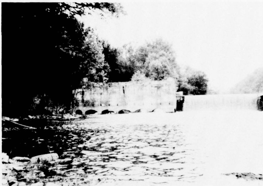
PHOTOGRAPH NO. 5 Outlets from Mill Structure
