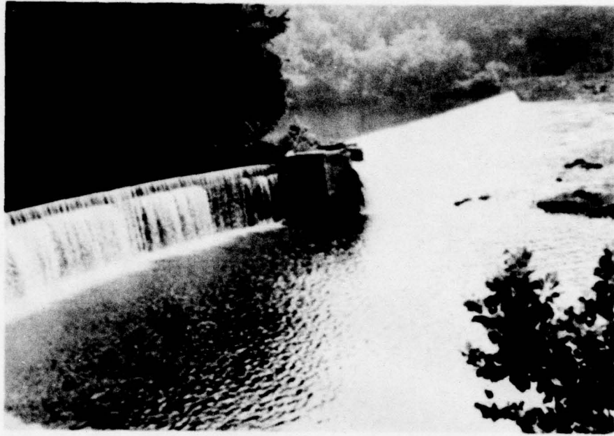
PHOTOGRAPH NO. 1 The Straight Spillway
