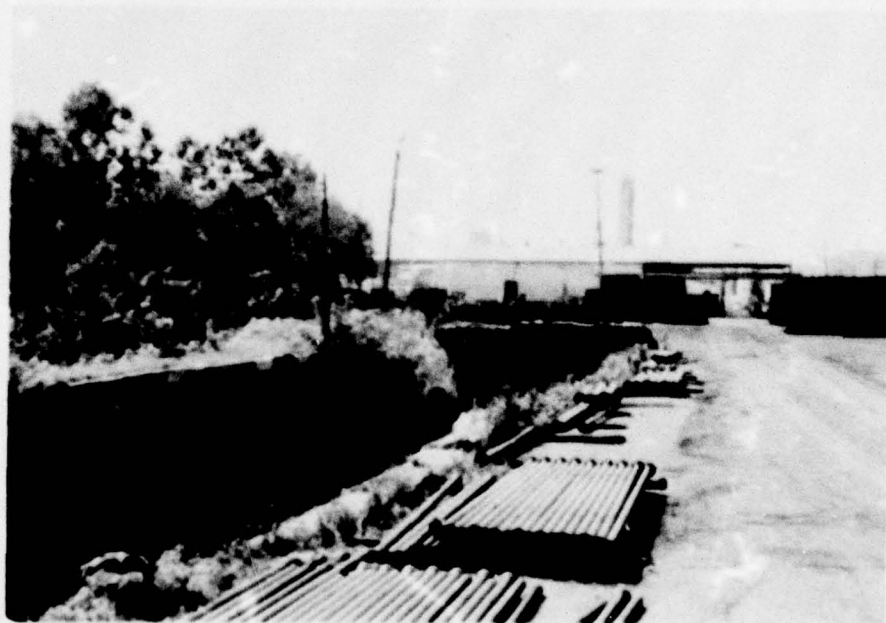
PHOTOGRAPH NO. 4 Griffin Pipe Company Plant on the Downstream Shore
