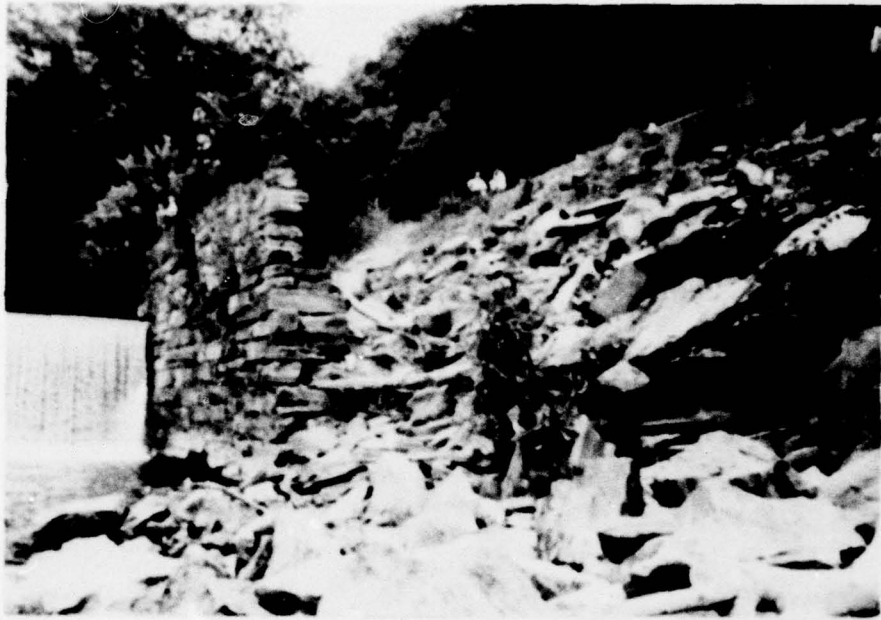
PHOTOGRAPH NO. 5 Left Abutment
