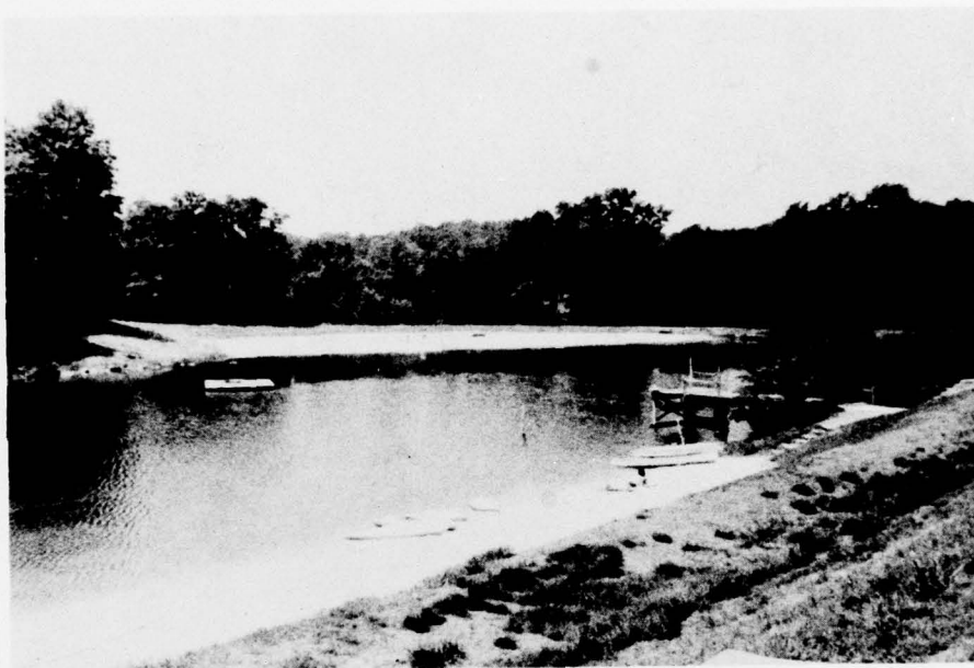
PHOTOGRAPH NO. 3 Emergency Spillway
