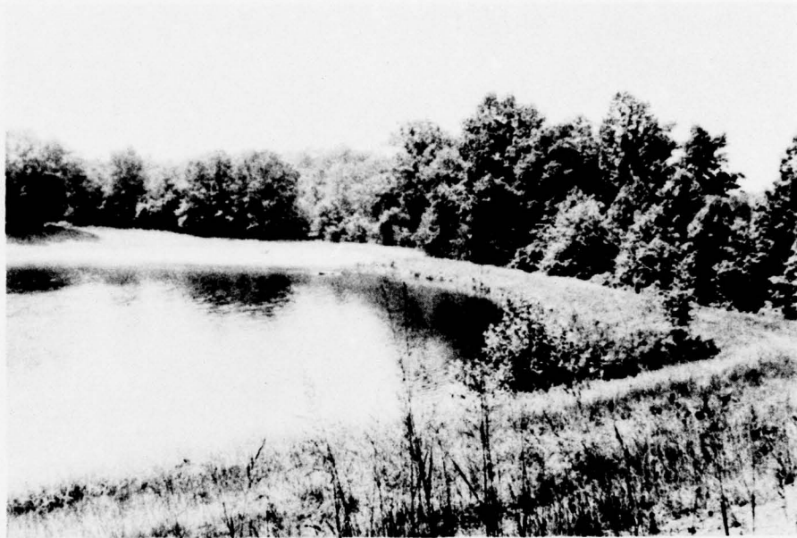
PHOTOGRAPH NO. 1 Upstream Face of Dam
