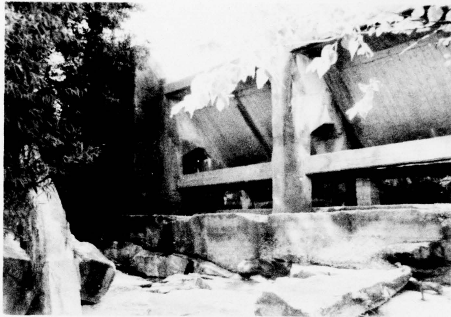
PHOTOGRAPH NO. 1 Right Abutment and Part of Concrete Structure
