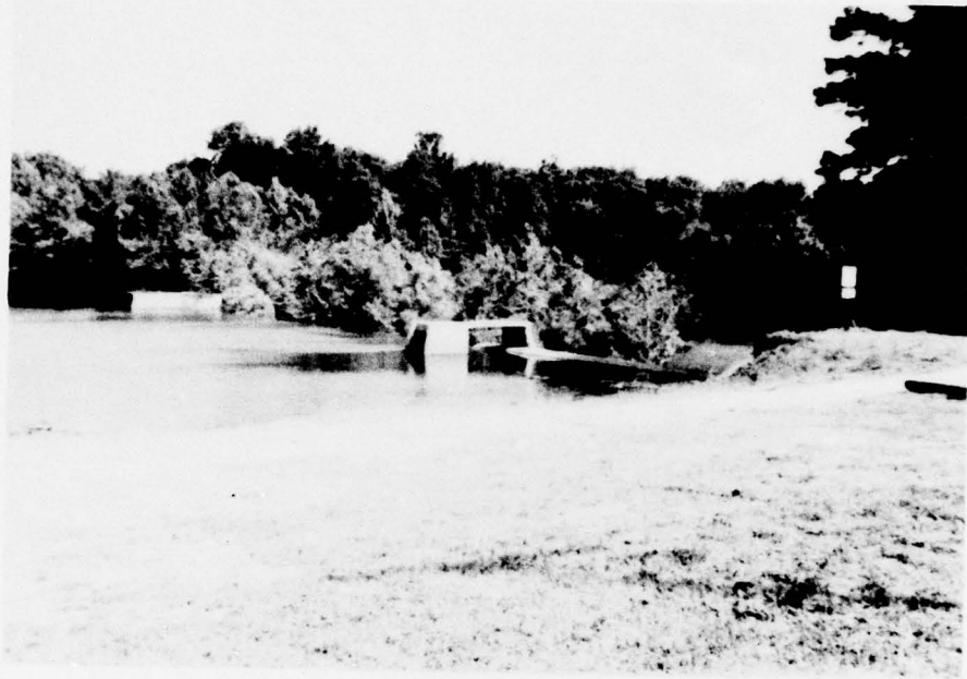
Overview of Dam
