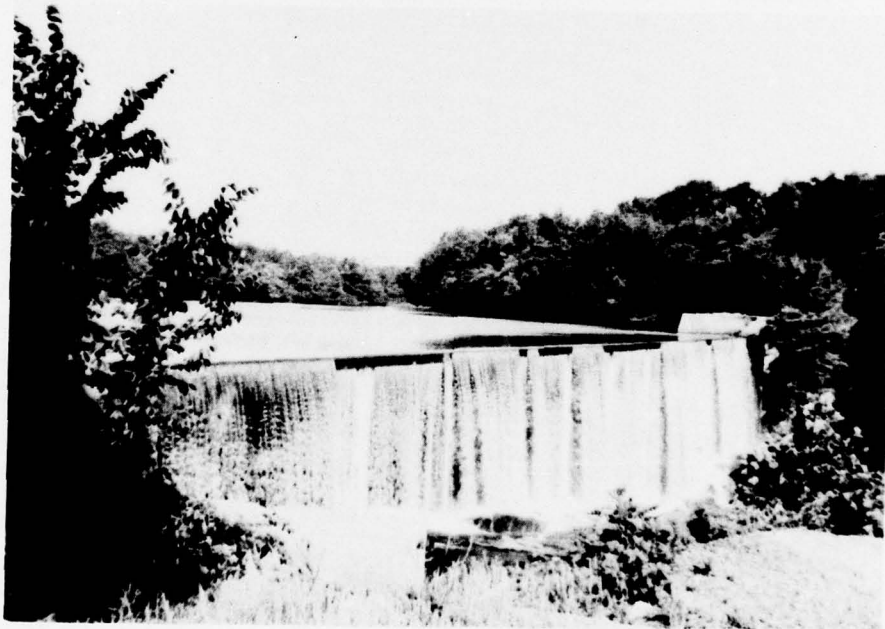
Front View of Dam
