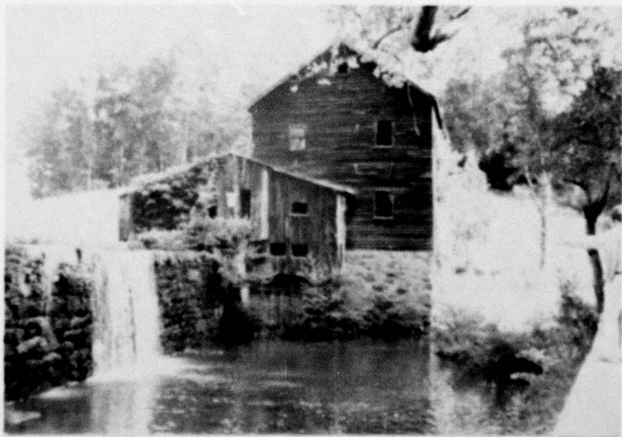
PHOTOGRAPH NO. 4 Old Mill House at Left Abutment
