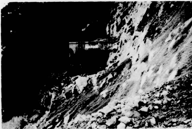
Figure 32. View of tunnel after earthquake
