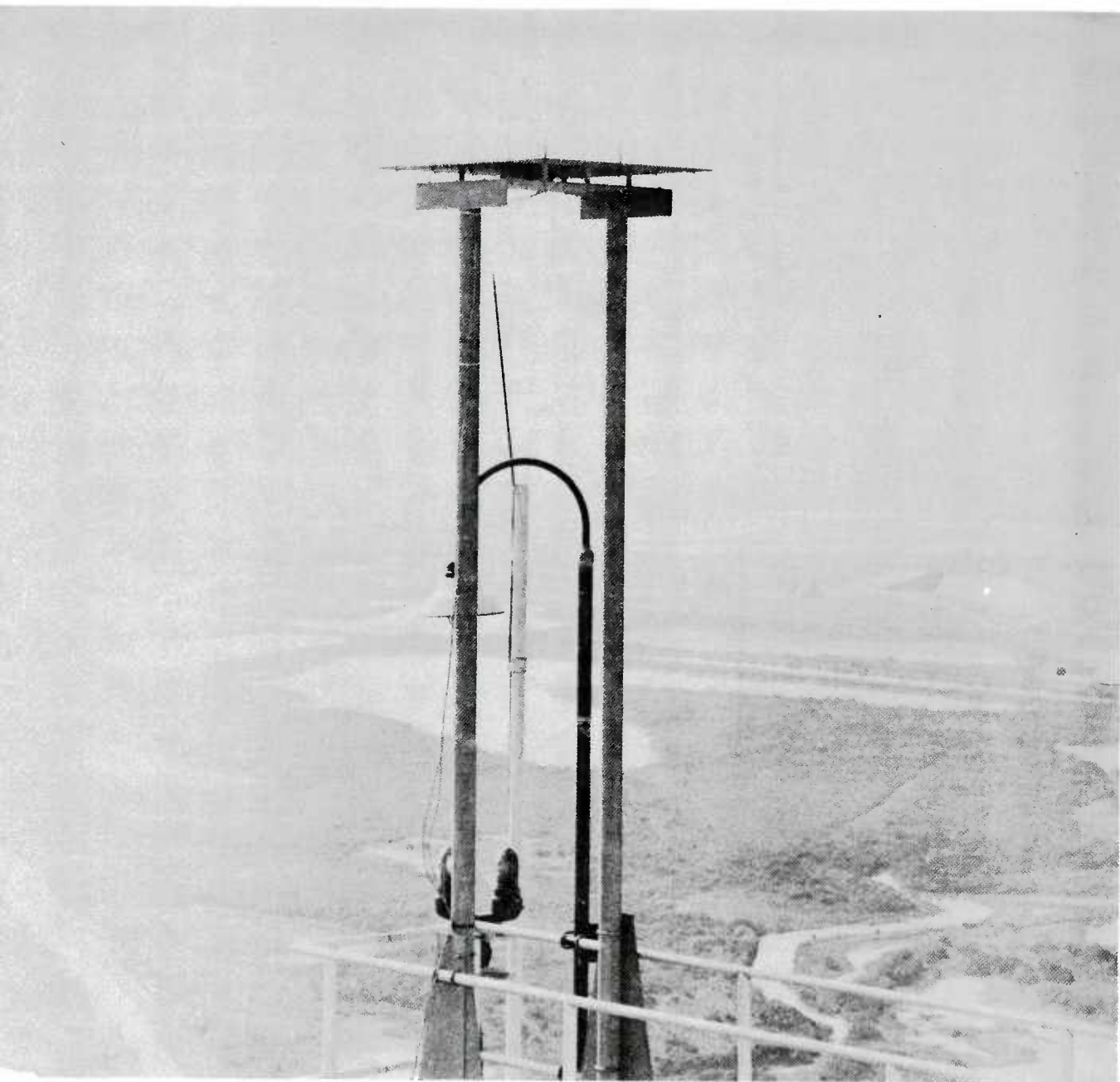
MOBILE SERVICE STRUCTURE, ARRAY #1
