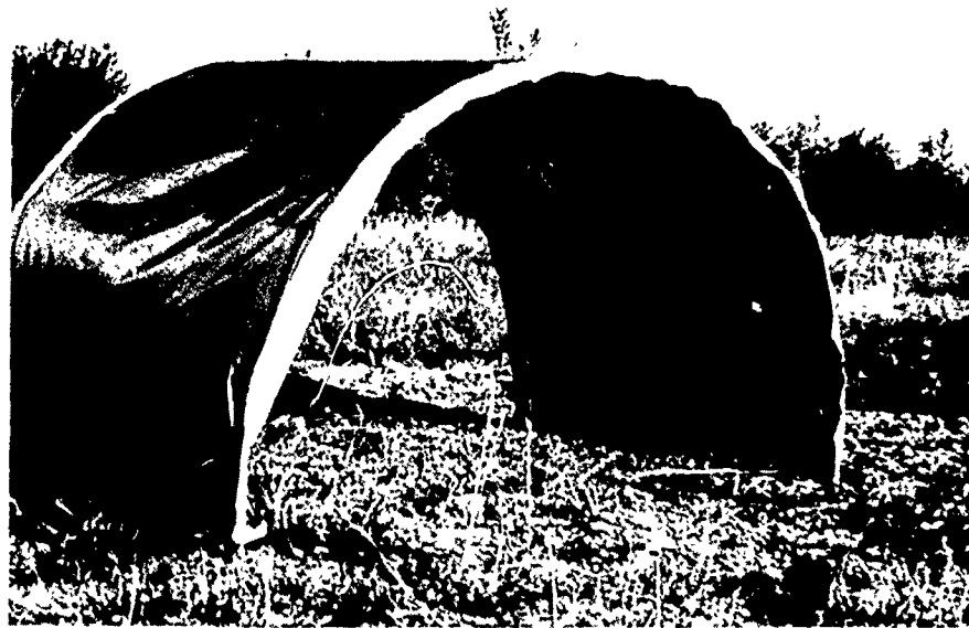
Figure 9. Tube frame with fabric in place.
