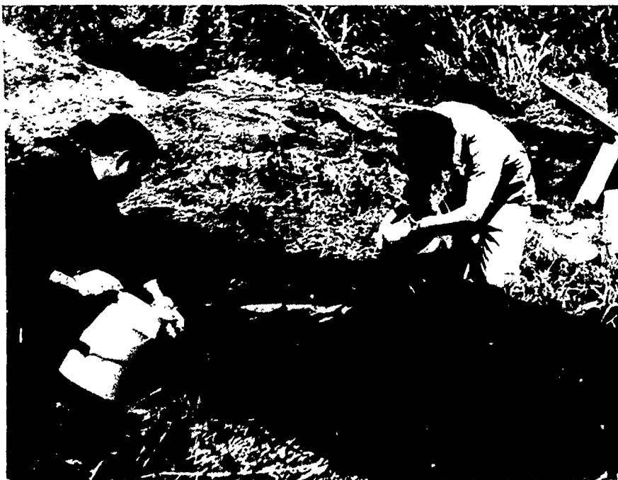
Figure 11. Introduction of foam at midlength of foam/fabric bag.
