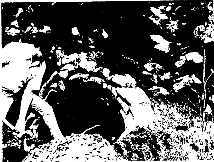
Figure 38. Adding soil cover to sandbag cover.
