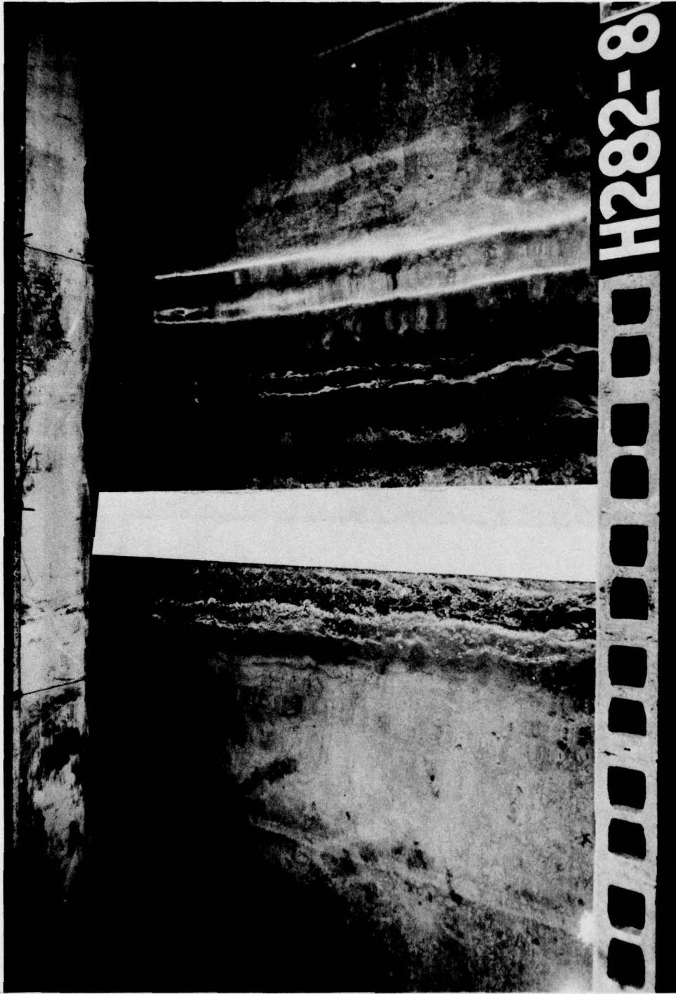
Photo 9. Overhead view of Plan 1 under attack of 3.0-sec, 2.0-ft waves
