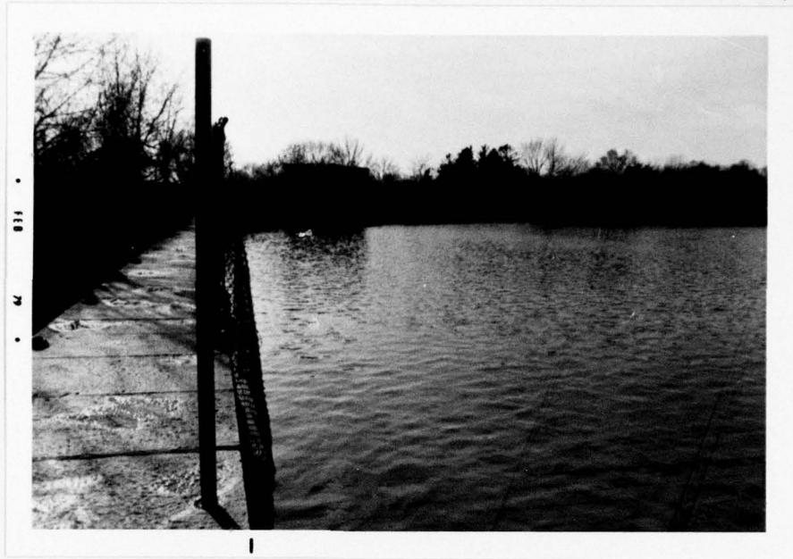
CREST OF NON-OVERFLOW MASONRY SECTION WITH "GATE HOUSE"
