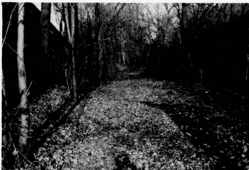
DOWNSTREAM TOE OF MASONRY SECTION
