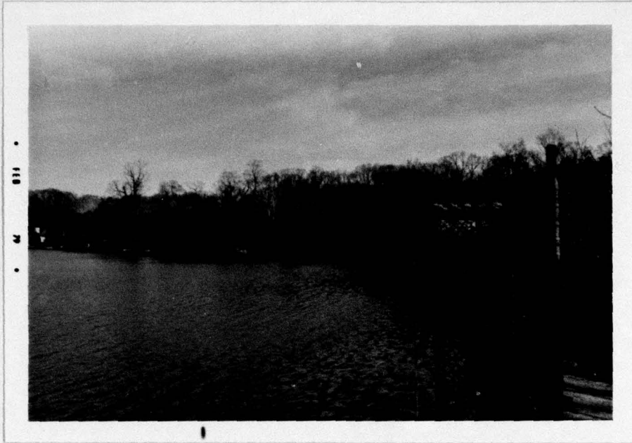
NEW ROCHELLE RESERVOIR No. 1 DAM OVERVIEW - NORTHEASTERN END
