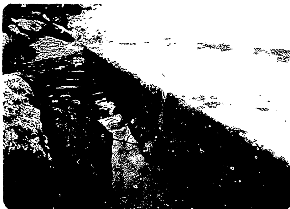
Undermining of Downstream Apron at Western End of Dam
