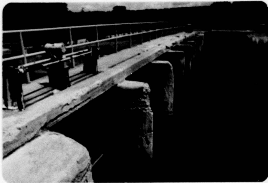
Deteriorated Concrete on Piers and Bridge Deck; also, Lifting Device Used for Raising Stopgates
