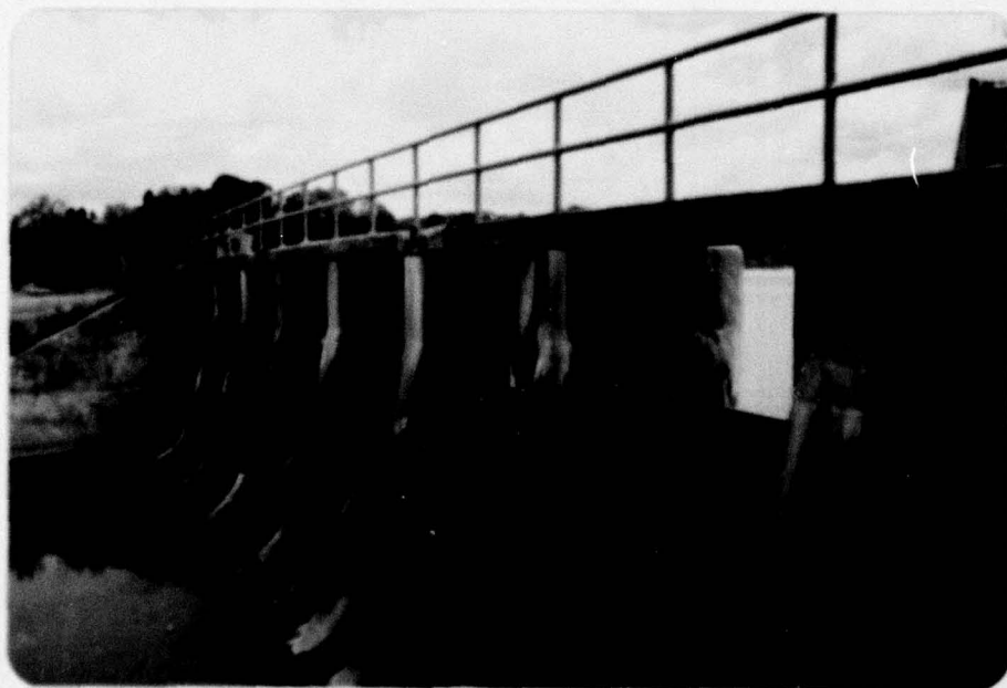
Spillway - Downstream Portion of Ogee Section
