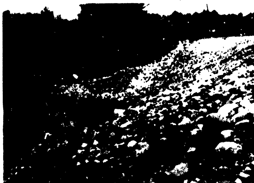
Downstream Slope of Reconstructed Segment of Dam Seepage Noted at Toe in This Area
