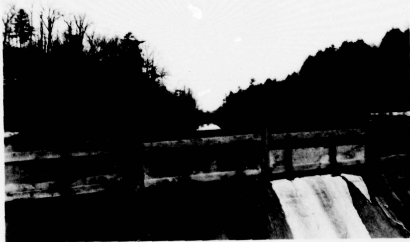
RESERVOIR @ DASHVILLE DAM
