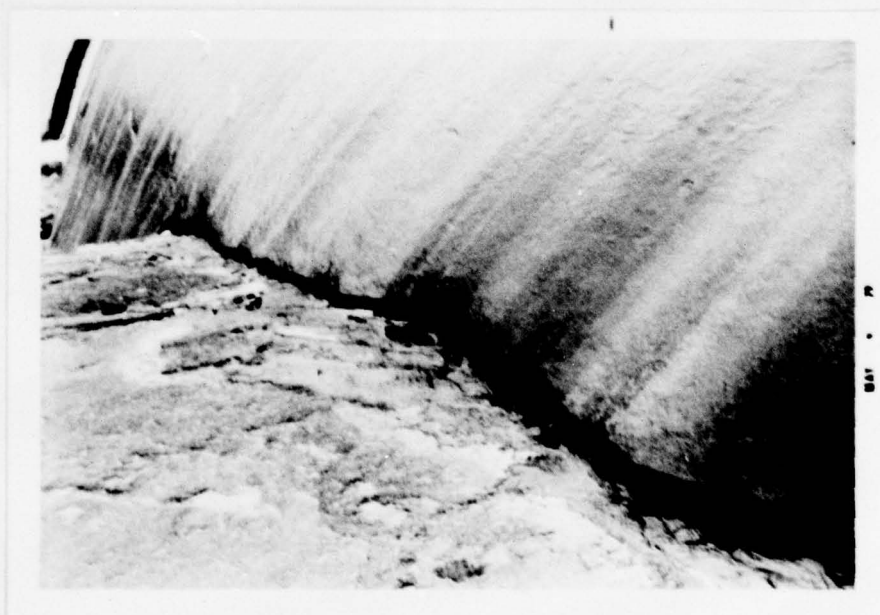
INTERFACE ALONG FOUNDATION AND NON-OGEE SPILLWAY SECTION
