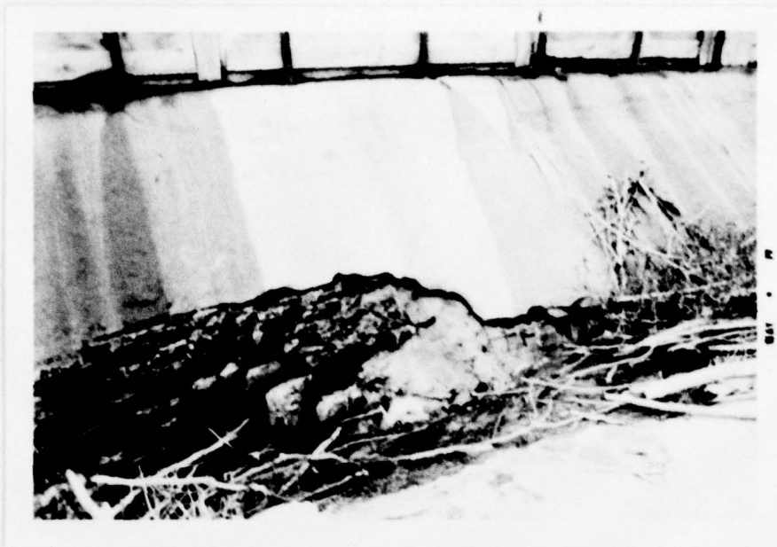
CONCRETE SURFACE SPALLING @ SPILLWAY
