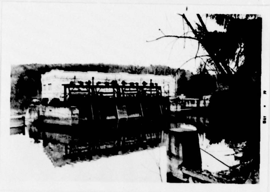
POWER STATION - UPSTREAM
