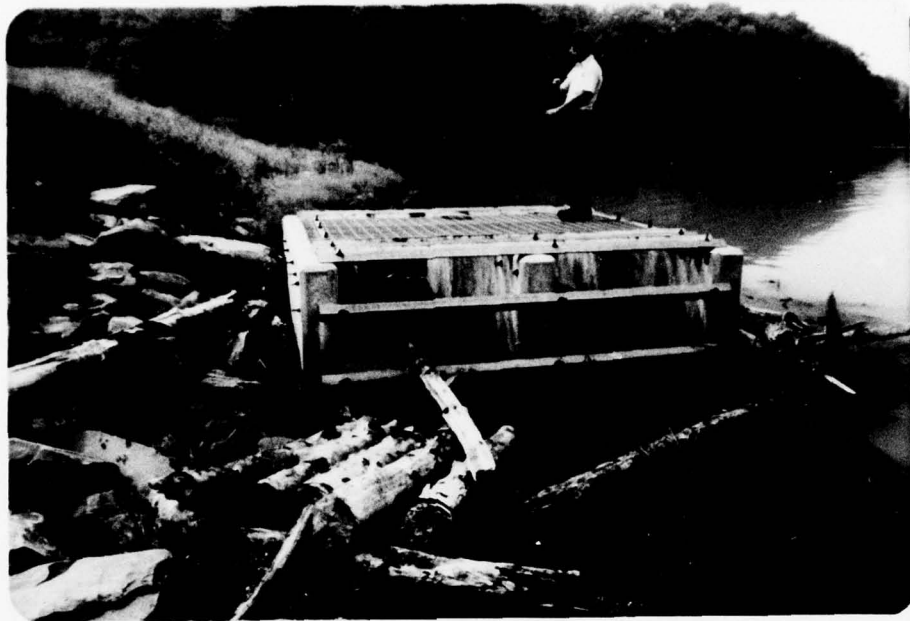
Left Side of Principal Spillway Riser Photo #4
