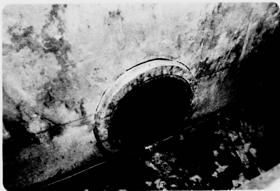
Outlet of 36" Concrete Pipe in Impact Basin Photo #7
