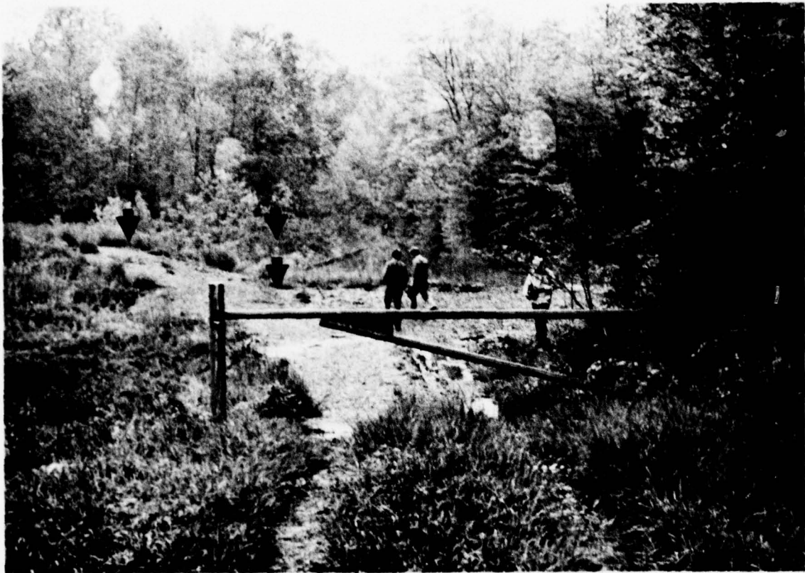
SPILLWAY IN RIGHT ABUTMENT (Outlined with Arrows)
