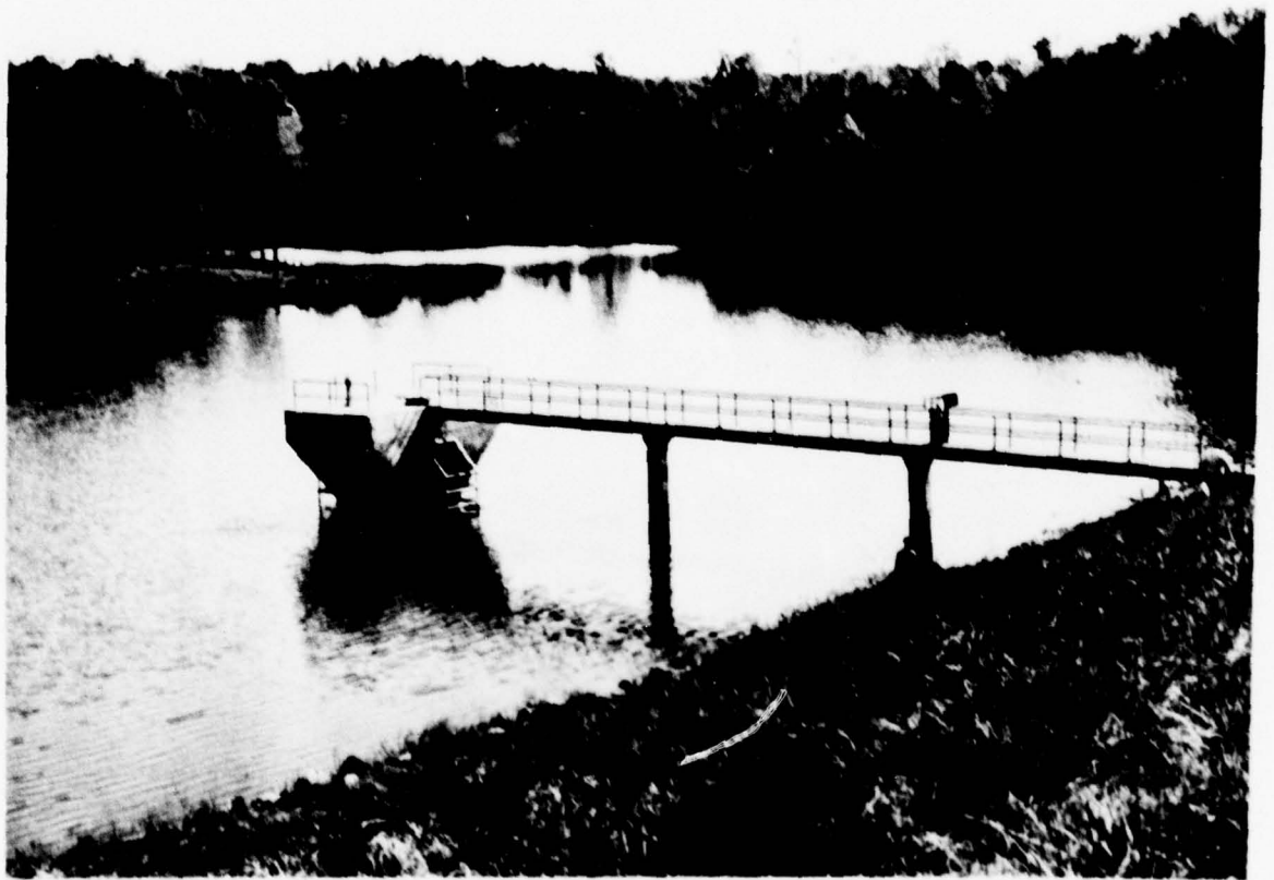
INTAKE STRUCTURE AND CATWALK Photo #2
