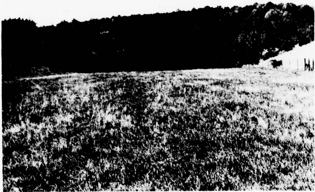
VIEW EMERGENCY SPILLWAY
