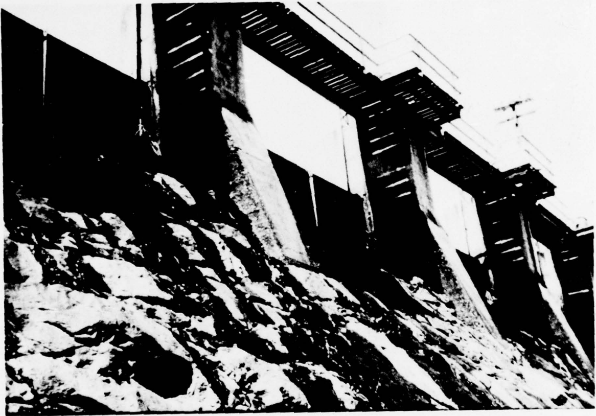
CLOSE-UP CATWALK AND GATE SECTION
