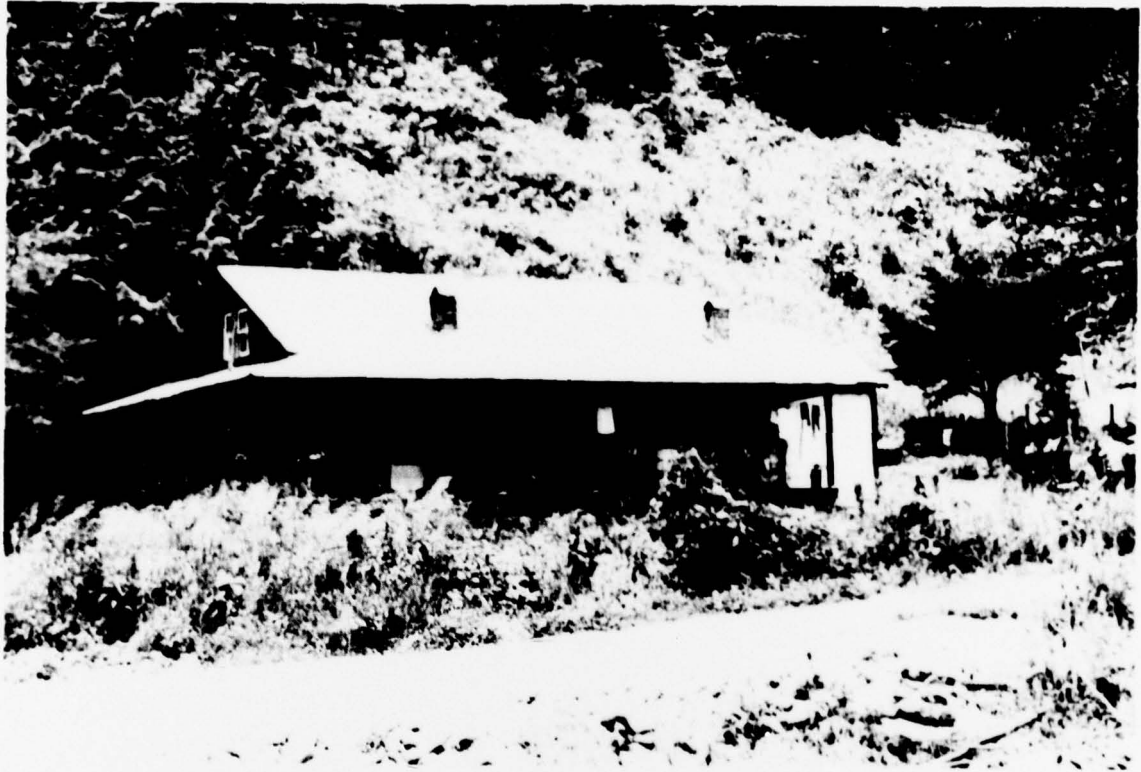
HOUSE LOCATED DOWNSTREAM IN FLOODPLAIN. THE SLOPE IN BACKGROUND IS TYPICAL OF SIDE SLOPES BETWEEN IMPOUNDMENT AND THIS HOME.
