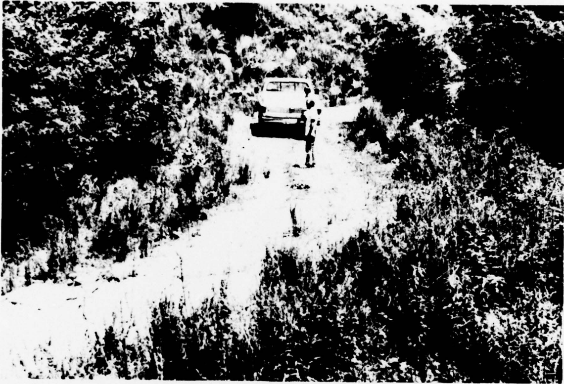
VIEW SHOWING HAUL ROAD ACROSS CREST OF DAM
